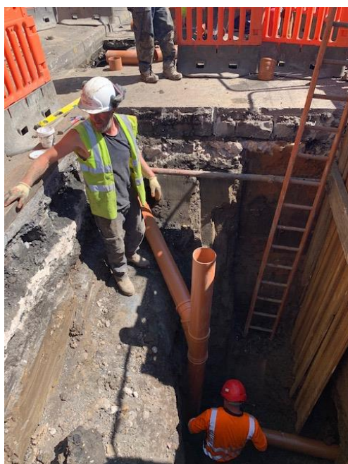
Drainage repairs on Hyde Rd outside B&M Store, Gorton
